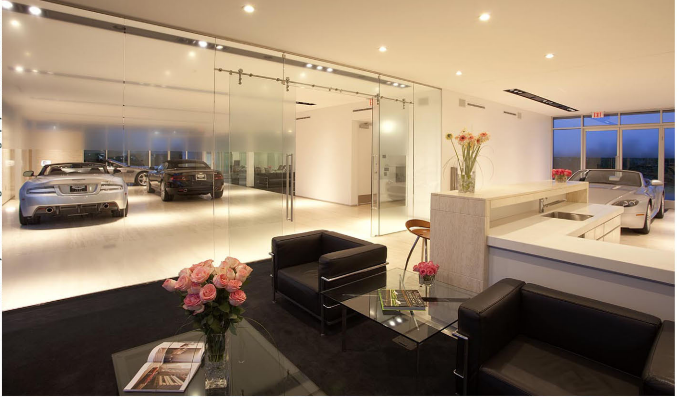
Inside, a glass wall that can be opened and closed was installed to section off parts of the showroom on special occasions. "A glass sliding wall was hung on rollers," said Tony Dellicolli, RA, President of Cityscape Architects. "The idea is that if they are having an exclusive showing of a car or a private party, they can close off two-thirds of the showroom and have an open bar. You never have exposure to anyone else in the showroom. It plays off the exclusivity."
