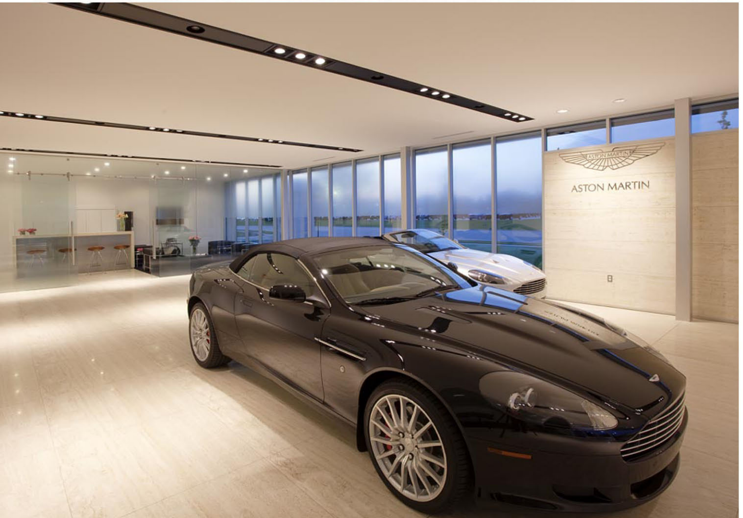
The travertine floor panels are backed with a steel plate so that they can sustain the load of the automobiles.
